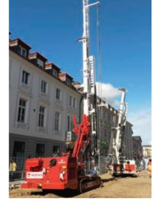
to reduce compressed air losses and dangerous blow-outs during NATM excavation. The permeability of the subsoil on a 2m-thick crown around the excavation area needed to be reduced in order not to exceed the limit of 1x10<sup>-7</sup>m/ sec. To obtain this, the use of low-pressure grouting had been envisaged by the designer. The permeation grouting was started in the autumn of 2014 by Rodio Spezialtiefbau, working as a subcontractor of BeMo/FCC.
