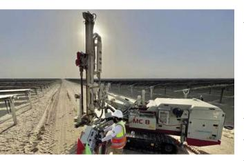
One of the two Comacchio MC 8 rigs being used to install the foundations for a solar farm in the UAE The Gulf Cooperation Council region has considerable renewable energy potential, particularly for solar photovoltaic (PV) generation. The United Arab Emirates (UAE) has managed to attract some large-scale solar PV projects, requiring highly productive and cost-effective drilling solutions for the installation of photovoltaic modules.
