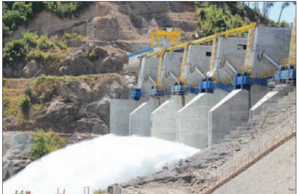
The Angostura hydroelectric power plant
