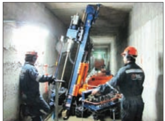
Working within the narrow galleries of the dam
