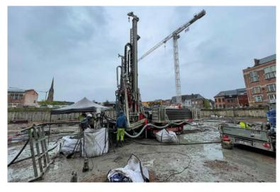
The ability of the Comacchio GEO700A drill rig to handle coarse gravel layers proved invaluable on a geothermal installation job for Belgian specialist Smeyers.
