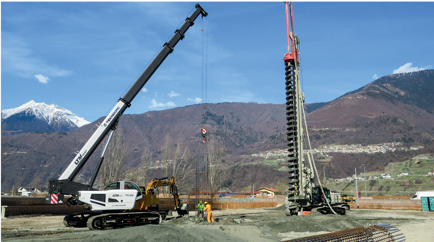
The reinforcement cage insertion phase
