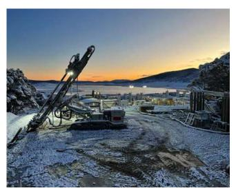
Grouting work carried out with the aid of a Comacchio MC 22 rig allowed tunnelling to continue on the Snowy 2.0 project after a shink hole developed stopping the TBM
