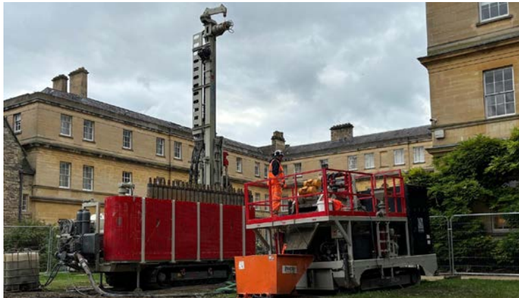
A Comacchio GEO 909 GT drill rig and An Elgin mud recycling system were employed by Rendesco for the creation of boreholes for a ground source heating project at Oxford's Trinity College
