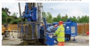
13-F, the F-Line has been expanded to handle greater diameters and drilling depths to meet the needs of customers working with vertical auger piles with up to 600mm diameter.
