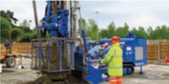
The F-line rigs – where F stands for ‘flight augers’ – are designed for the installation of mini piles using solid stem and continuous flight augers (CFAs). The first model of this series, the MC 6-F, was introduced to the UK market in 2016, with the first unit supplied to foundation engineer Roger Bullivant.
