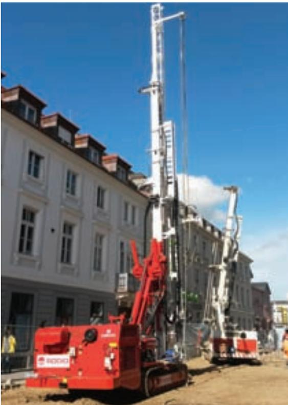
to reduce compressed air losses and dangerous blow-outs during NATM excavation. The permeability of the subsoil on a 2m-thick crown around the excavation area needed to be reduced in order not to exceed the limit of  $1 \times 10^{-7} \text{m/sec}$ . To obtain this, the use of low-pressure grouting had been envisaged by the designer. The permeation grouting was started in the autumn of 2014 by Rodio Spezialtiefbau, working as a subcontractor of BeMo/FCC.
